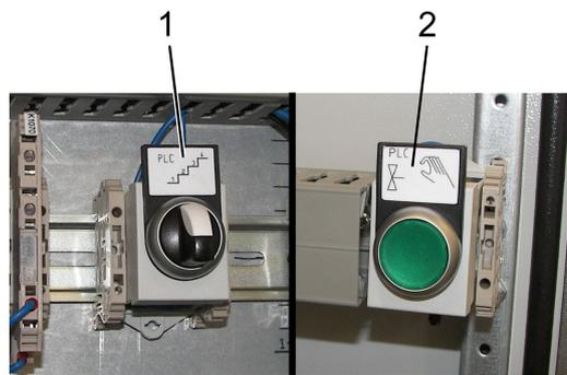
Figure 3.2-6: Service-pushbuttons in the control box
